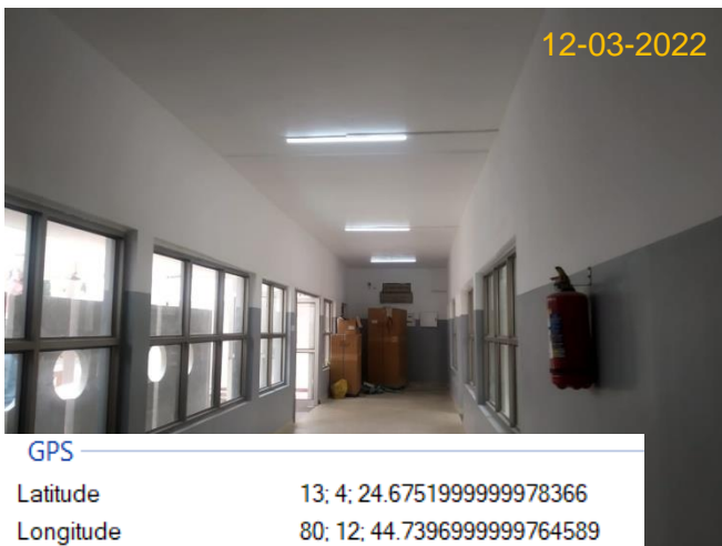
LED Batten Installed in Corridor
